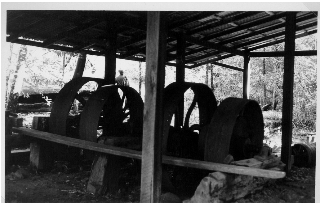
View inside sawmill showing large wheels for belt drive to machinery
