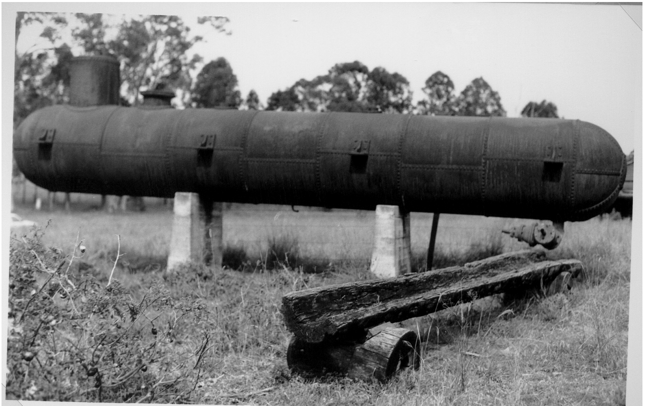
View of former sawmill boiler in use for molasses feed storage
