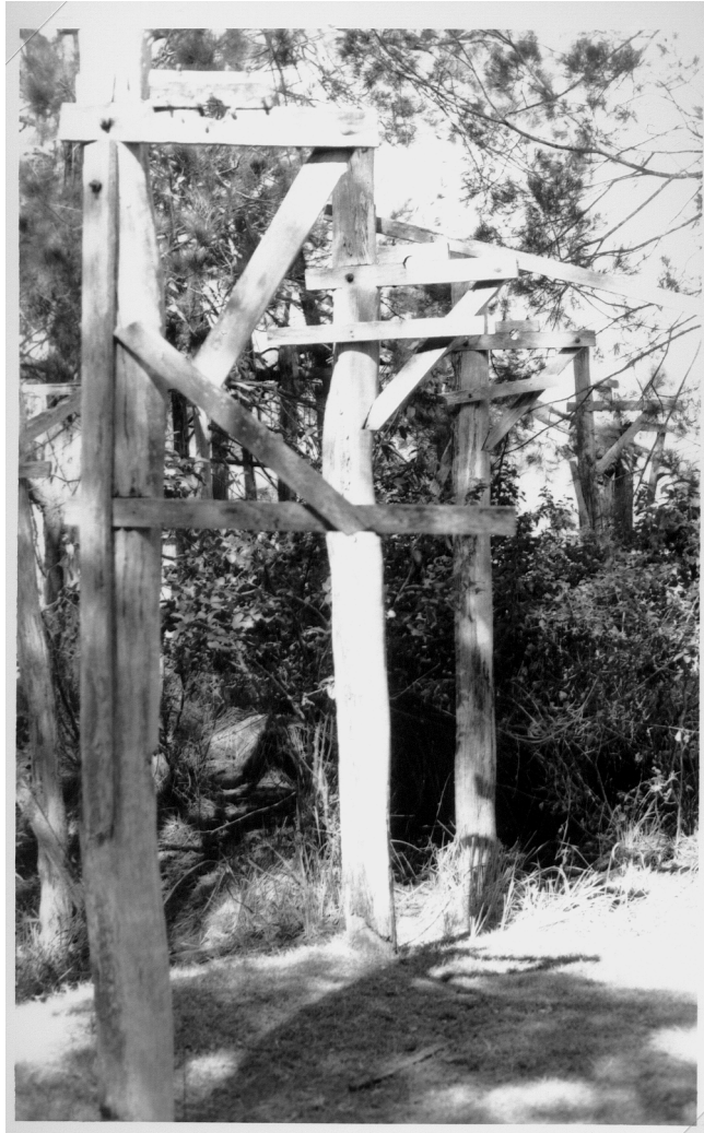
Series of main posts of sawmill shed with fittings for pulleys and belt drives
