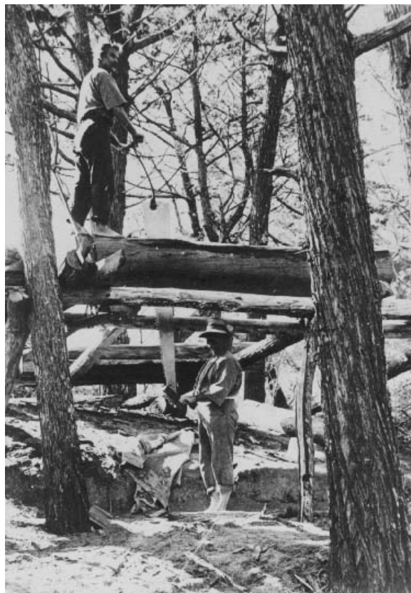
Pitsawing (unknown location).
