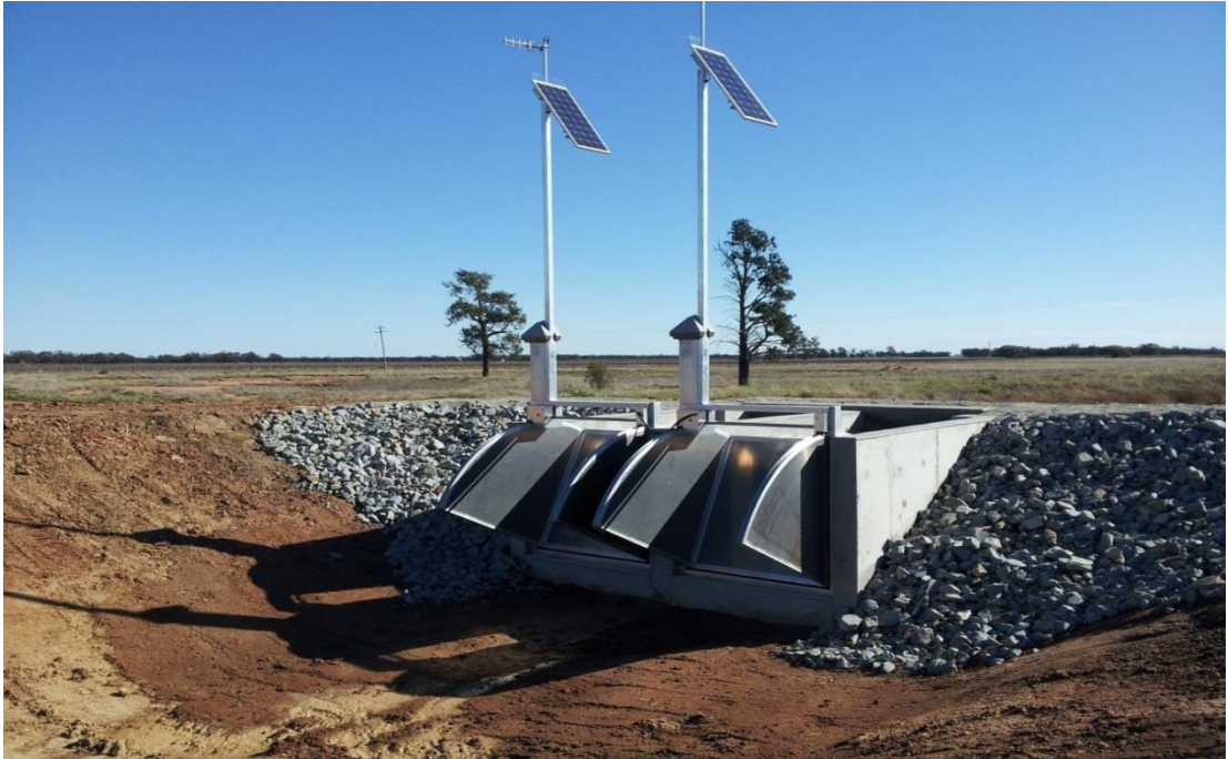
New TCC Regulating Structure on Kerarbury Channel (SP3)
