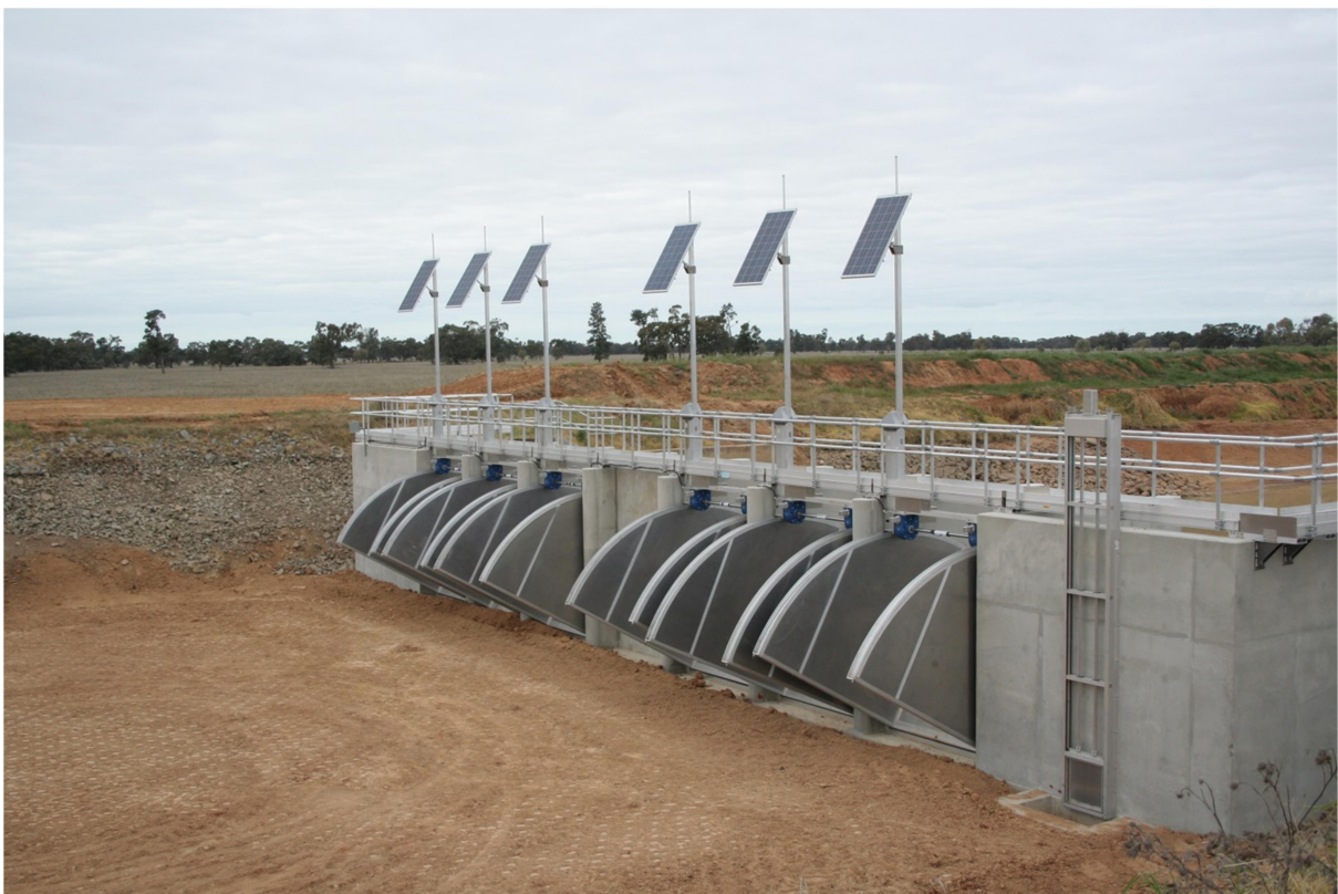
Photo 4 – One of three newly constructed regulators on CACL's Main Canal (SP 7)
