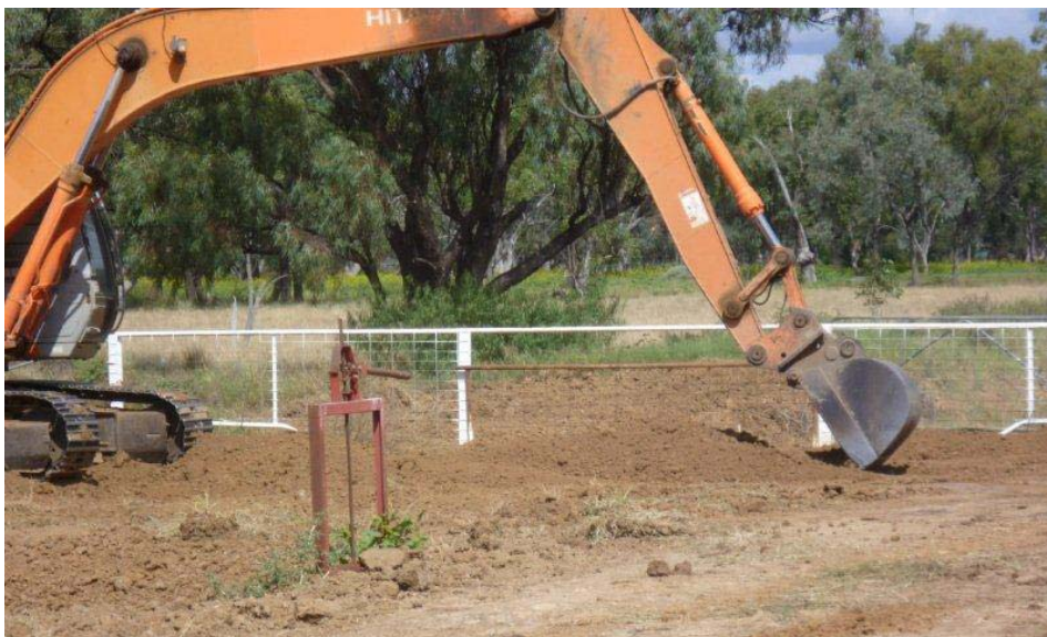
Photo 8. Local contractor, Marty Oriel, adding the final touches to complete the backfilling of the decommissioned channel in “Little Blacketts”.
