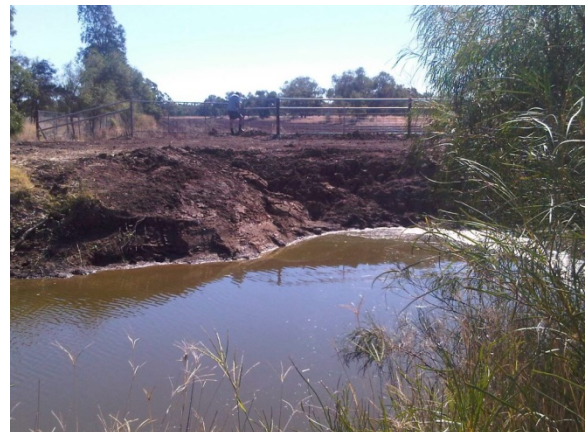
Photo 4. MIS outlet gates at Merenele Weir before (above) and after (below) decommissioning and back filling.
