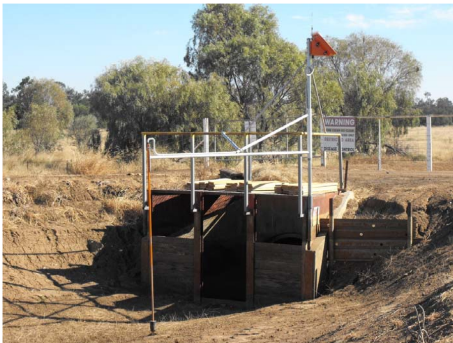
Photo 14. North Branch weir and channel depth gauge.
