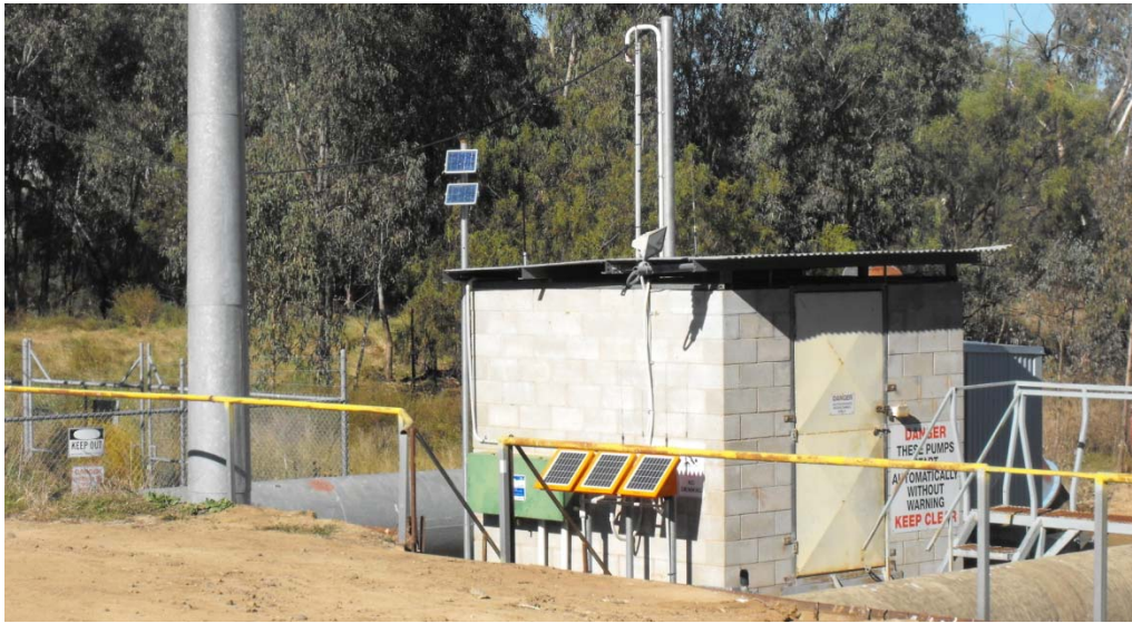
Photo 15. MIS Pumpshed and new telemetry base station including the 3 new C2e base station units (orange boxes) for data recording.
