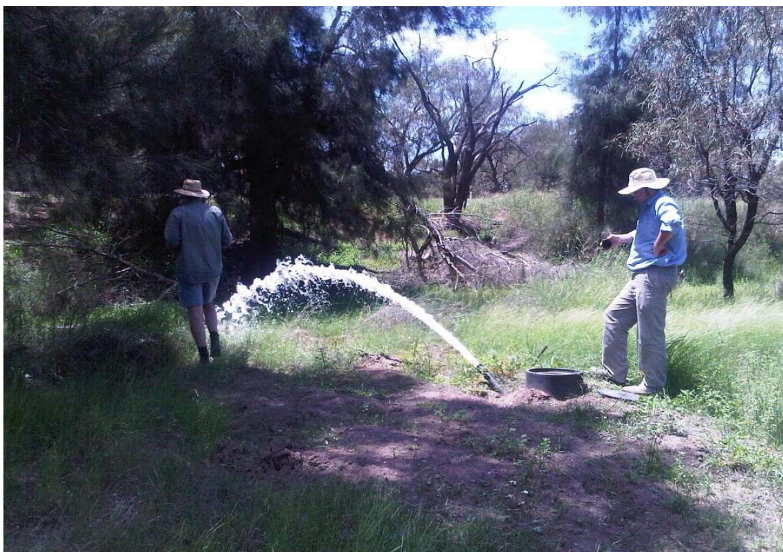
Photo 13. Mark Robertson from Darling Irrigation flushes the pipeline at the Bullagreen Creek scour valve, 30 km downstream of the pumps during testing of the pipeline, with Chairman, Nick Brennan.
