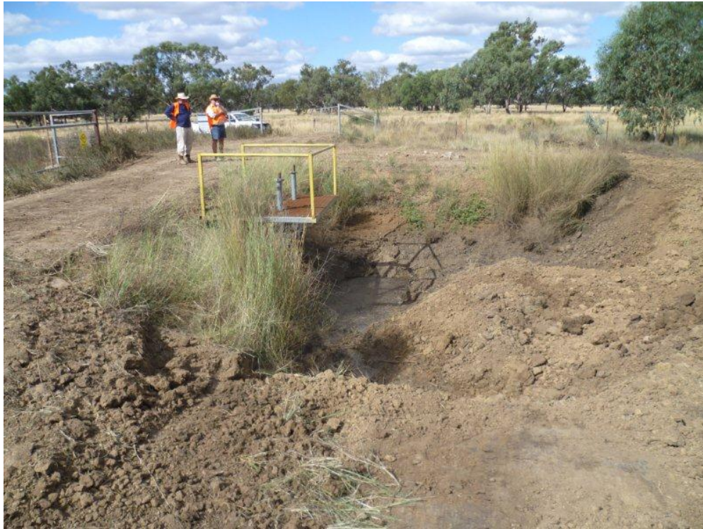
Photo 4. MIS outlet gates at Merenele Weir before (above) and after (below) decommissioning and back filling.
