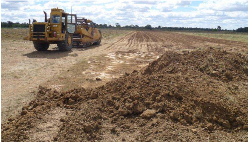
Photo 7. Local contractor, Kulkine Trust completed the filling in and compacting of the supply channel with an elevating scraper. Photo of channel in “Little Blacketts” after it was filled in.
