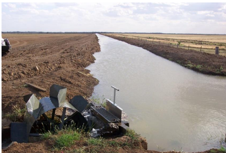
Open channel with Dethridge Wheel outlet prior to decommissioning
