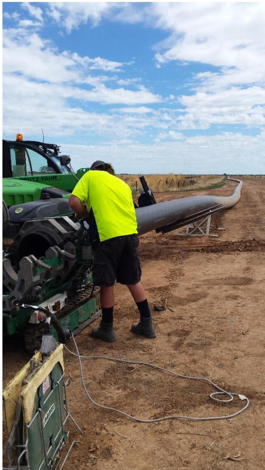
Pipeline welding
