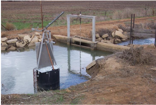
Pipe outlet and regulating structure prior to decommissioning
