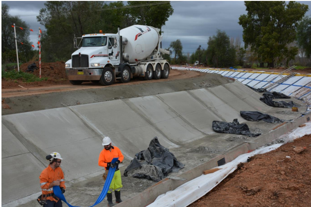
Local contractors using 7 cubic metre truck to deliver concrete to LVBC re-lining sites
