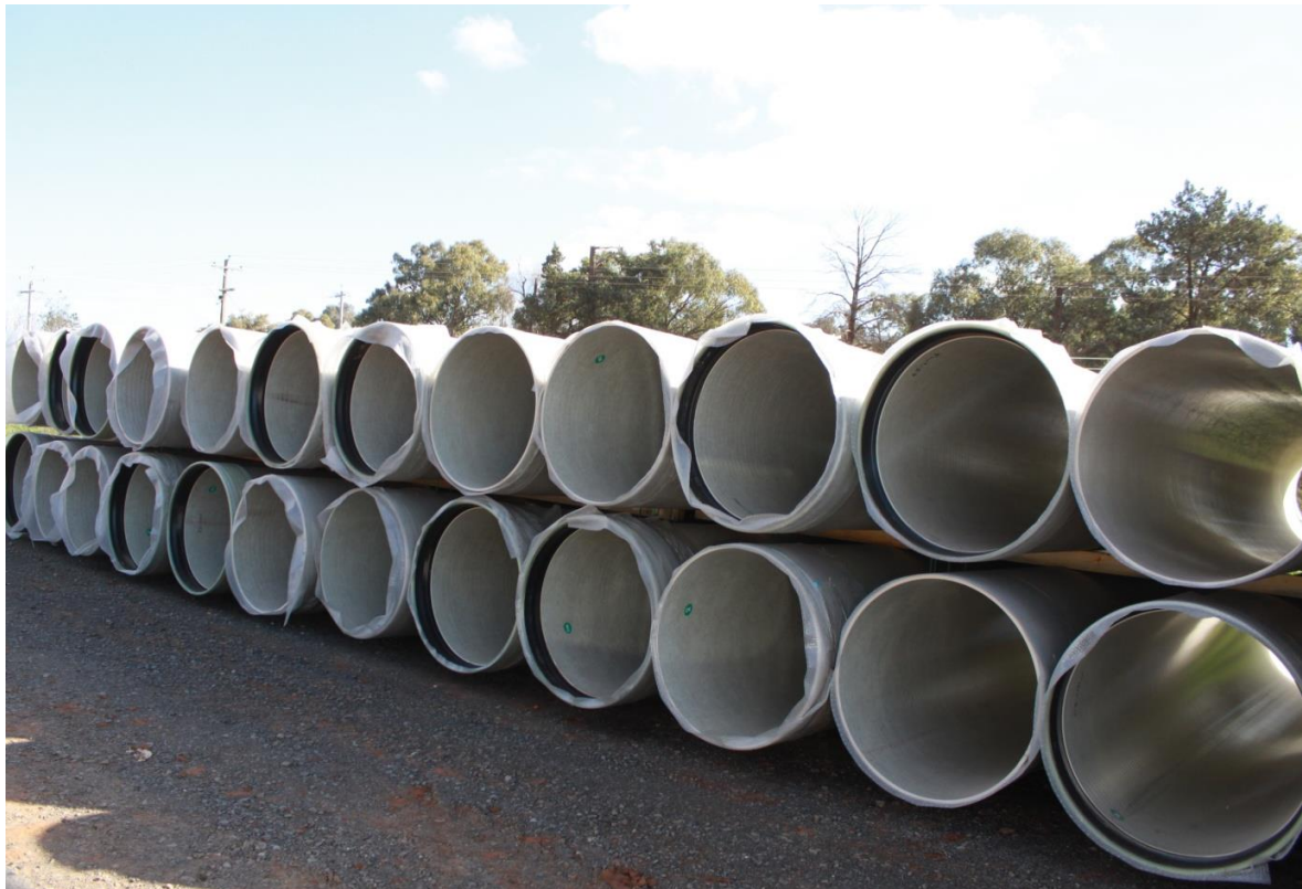
900 mm Glass Reinforced Pipes (GRP) in temporary storage close to construction site
