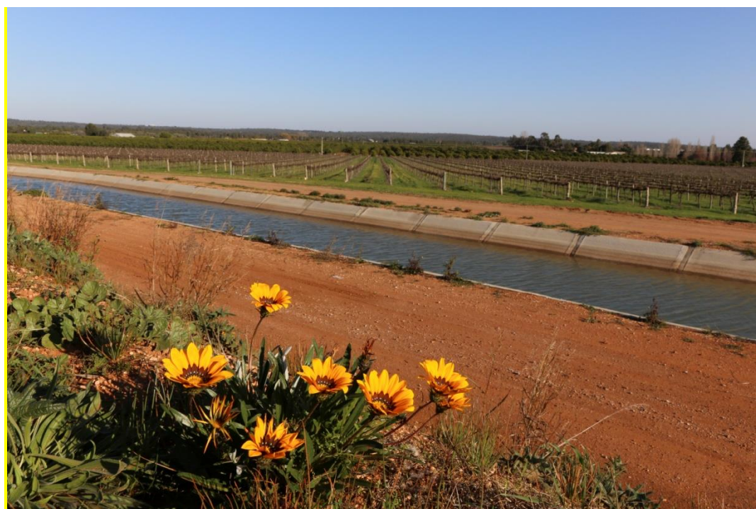
Section of the LVBC reinstated after relining works
