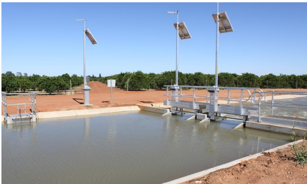
Remote Monitored Metered Outlet and Automated Regulator on LVBC
