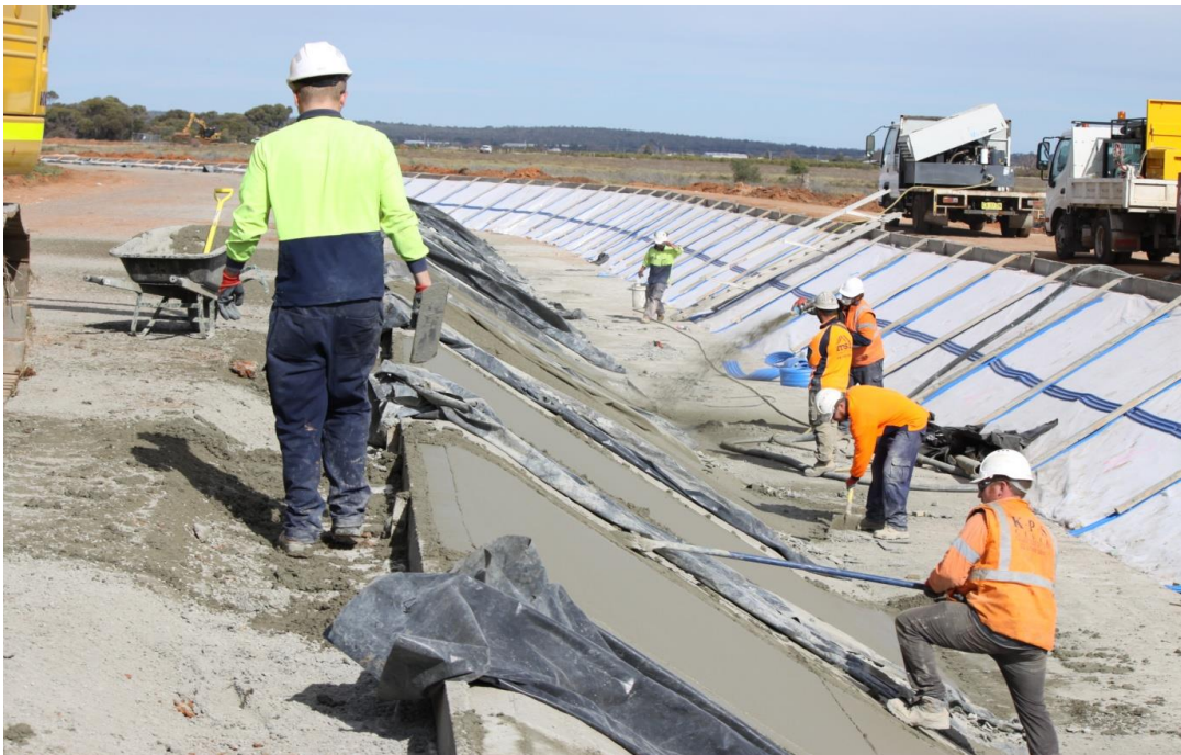
Formwork and Relining of the LVBC
