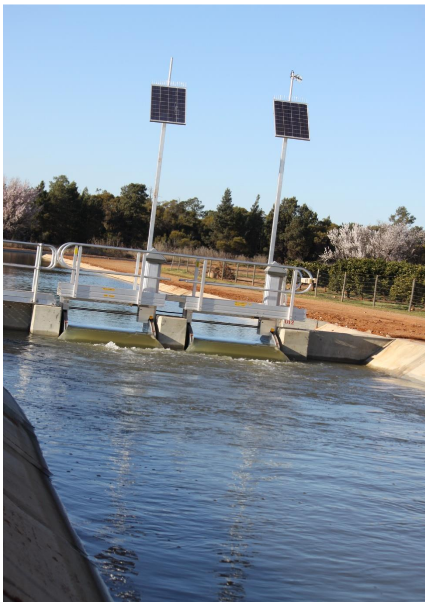
New Lake View Branch Canal regulator with automated gates
