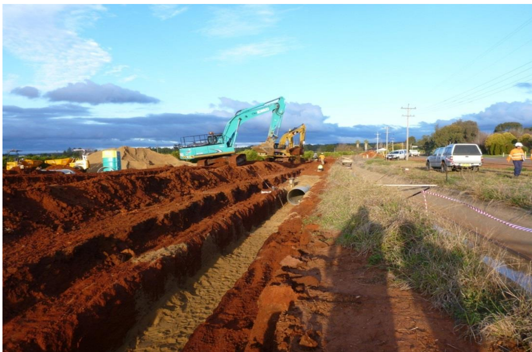
Installing Ballingal Branch Canal pipeline
