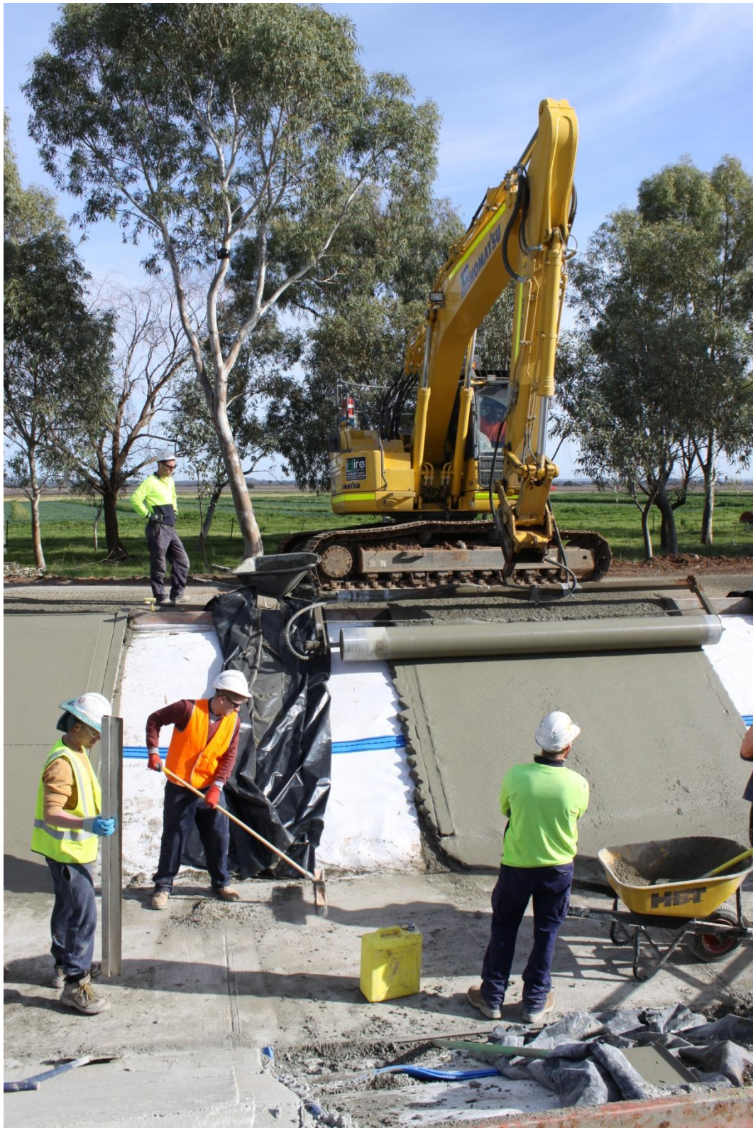
Innovation: Hydraulic driven Screeding Roller developed and used to increase productivity and reduce WH&S Risks to Employees
