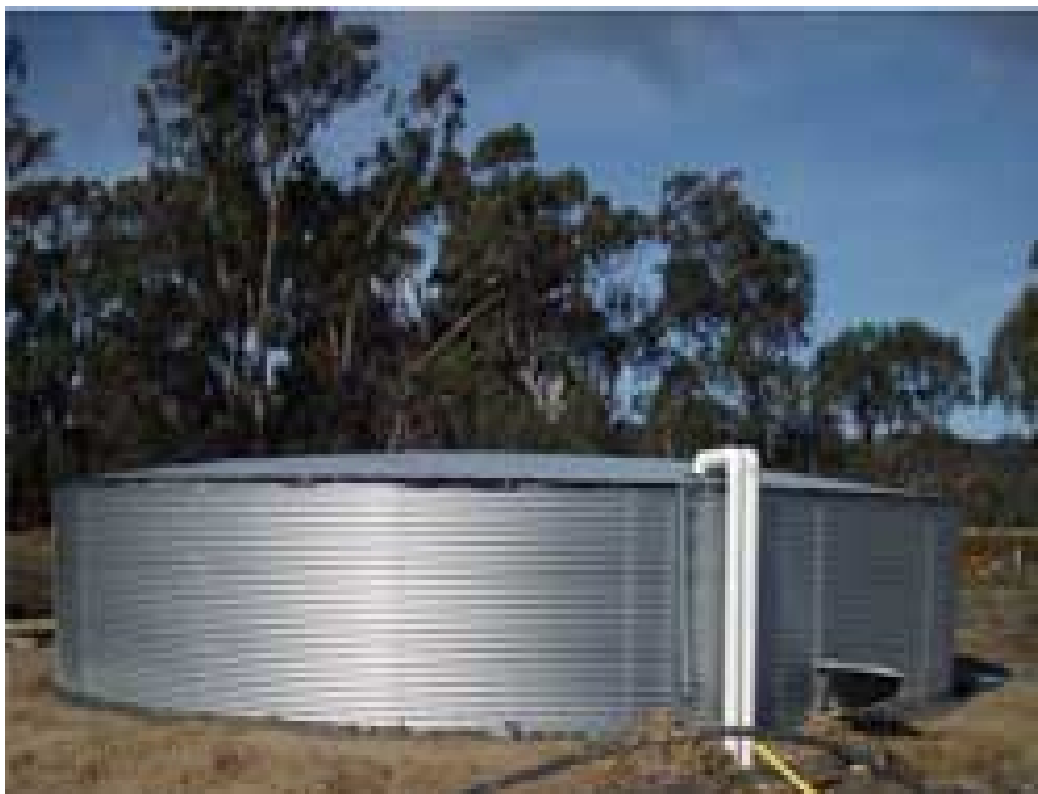
Photo 4 Typical 120,000 litre main header tank installed on 'Gundooi'
