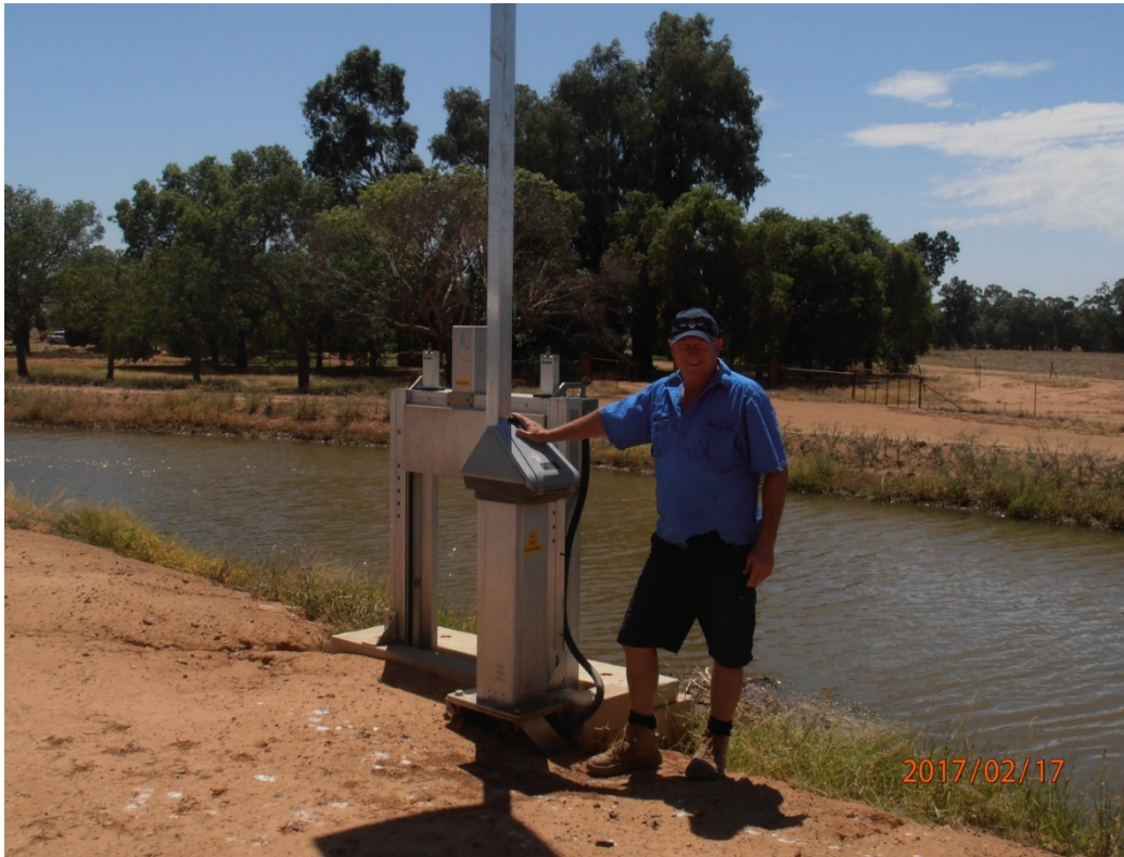
Photo 6 Martin McKinney at one of his new farm outlets—capable of delivering over 30 megalitres per day
