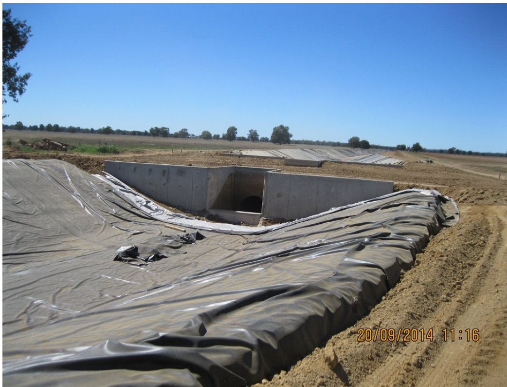
Photo 10 New channel crossing and liner installation upstream of 'Myall Plain'
