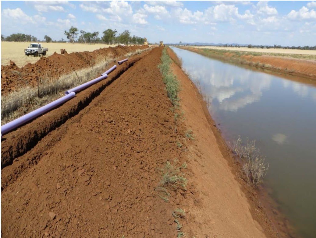
Photo 12 Construction of the stock and domestic pipeline by Mitchell Water
