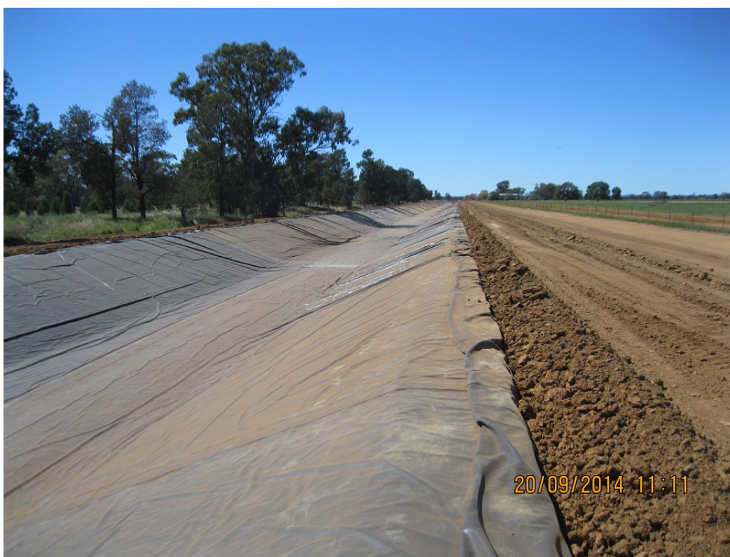
Photo 11 Completed liner installation at 'Myall Plain'
