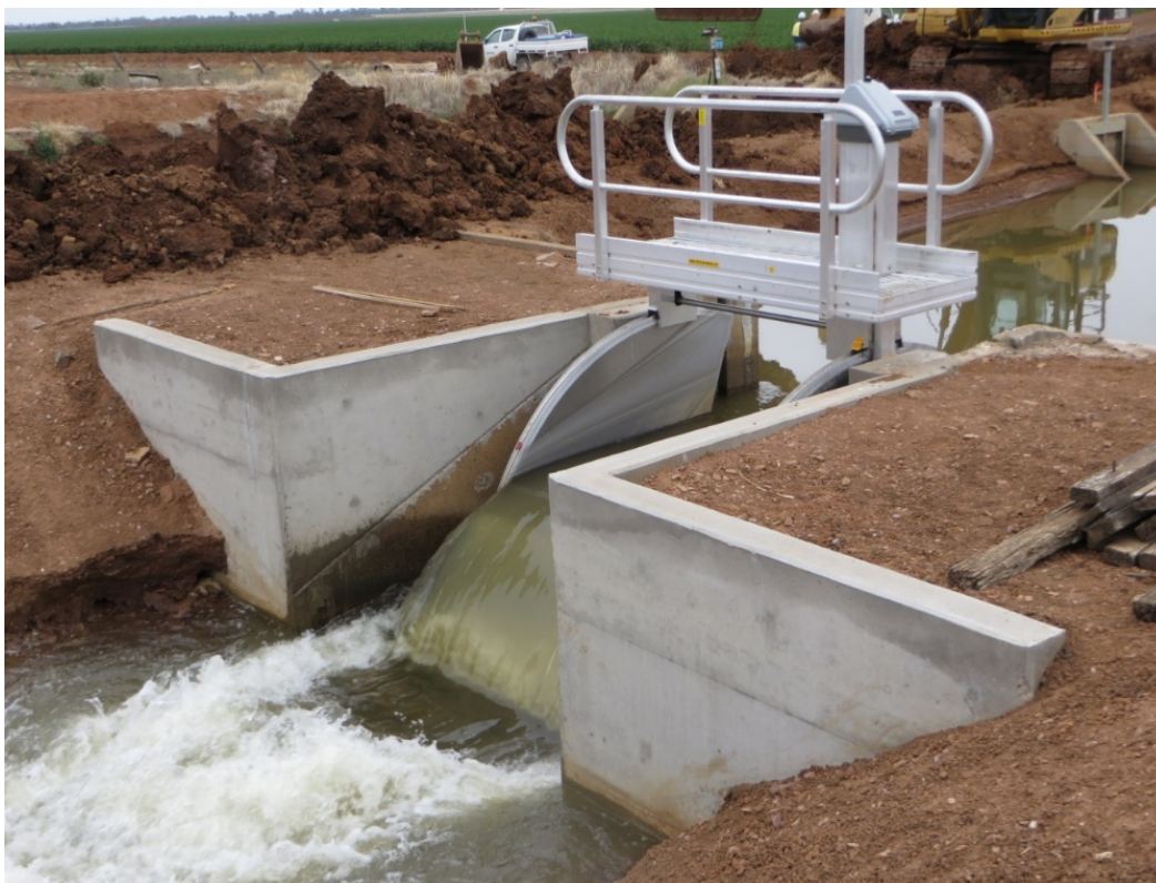
Photo 13 Newly installed flume gate regulating structure, with farm outlet in the background
