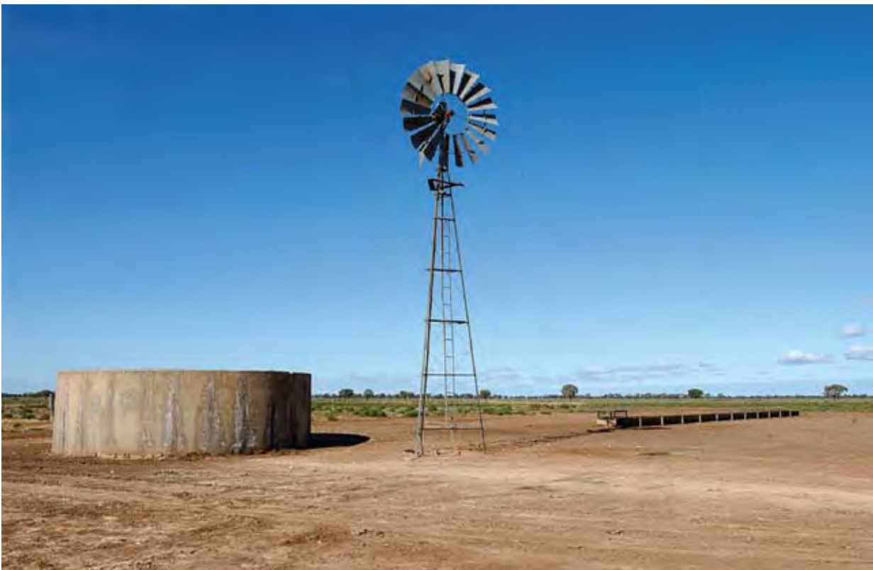
Windmill pumping groundwater for stock in Australia
