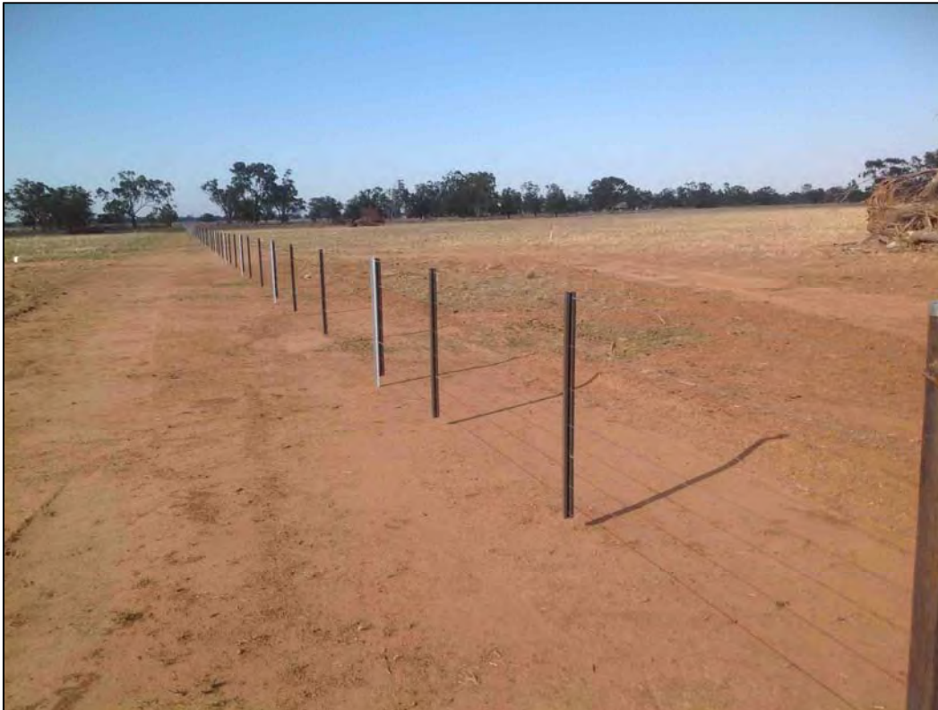
Figure 24: Example of a 'Weston' fence assembly. The design of each section was determined in consultation with landholders and intended agricultural usage.
