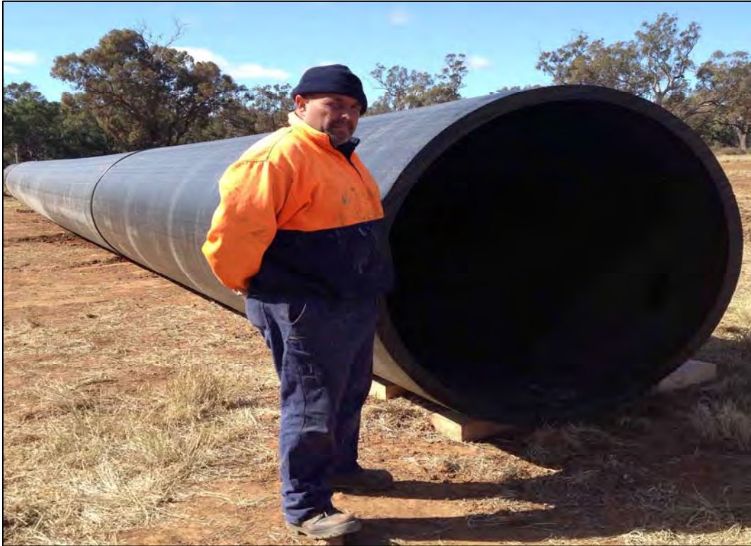
Figure 8: Bobby Sal from Irribiz Griffith, standing alongside Siphon 2 prior to installation. Constructed of 1600 mm diameter HDPE pipe, Siphon 2 traverses 392 m over the Travelling Stock Reserve, Ewenmar Creek and adjoining flood plain into 'Methalibah'.
