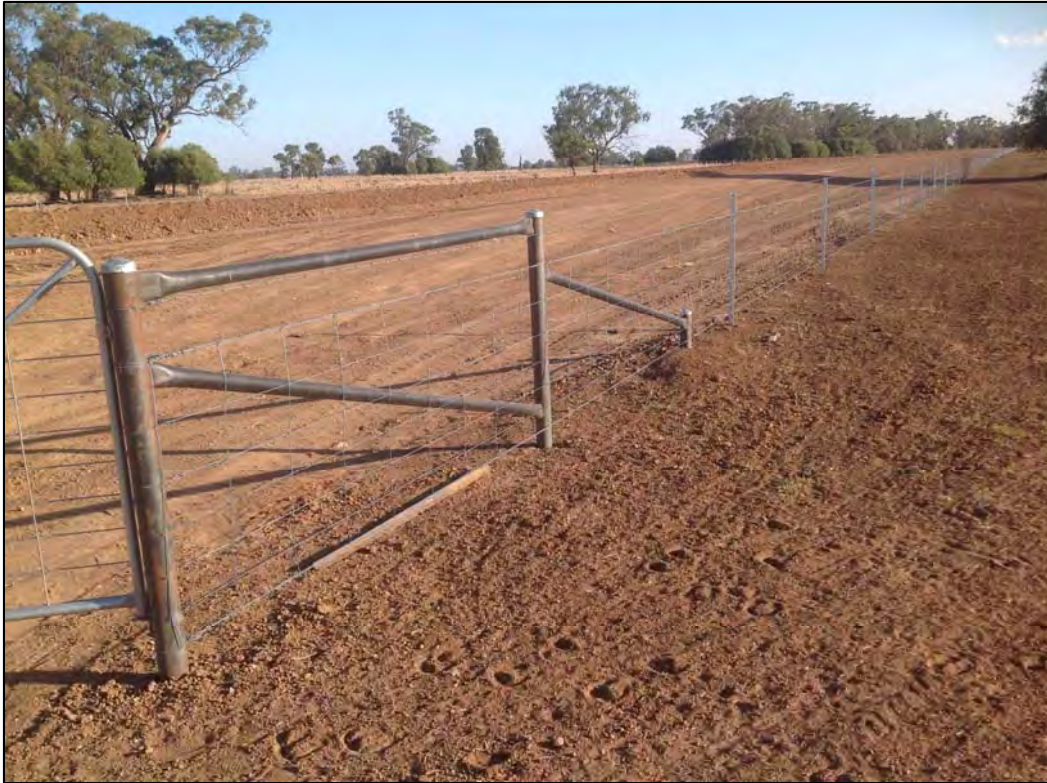
Figure 23: Approximately 25 km of fencing – such as this hinge joint fence and end-assembly – was constructed along new or decommissioned sections of channel.
