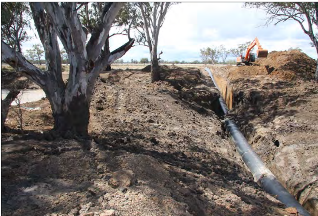
Figure 9: Siphon 3 transfers water from the Bottom Scheme channel beneath Ewenmar Creek, which was enclosed in a cofferdam (left) during construction, on 'Gillendoon'.
