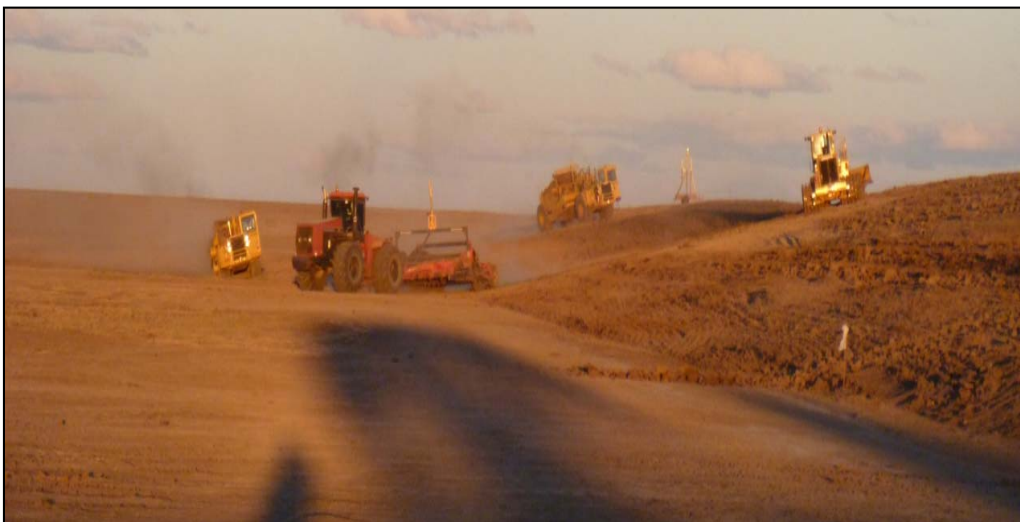
Figure 31: Construction operations of 'Milawa' on-farm efficiency sub-project
