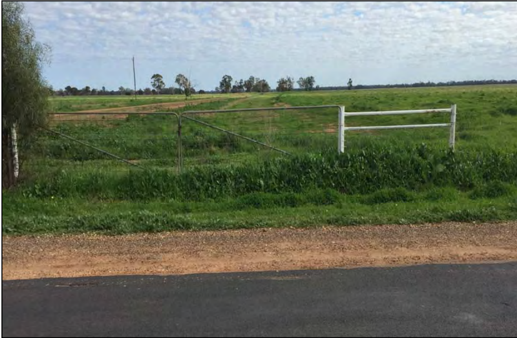
Figure 39: Looking west across the decommissioned Quambone Road crossing and along the decommissioned Scheme channel in “The Cedars”, approximately 60 km downstream of the Tenandra pump site.
