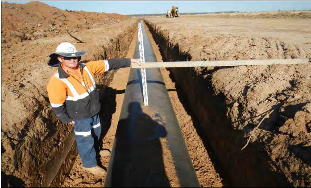
Figure 11: Quality assurance procedures on Siphon 1, including checking depth of pipe to ensure a minimum cover of 600 mm over the 800 mm HDPE pipe.
