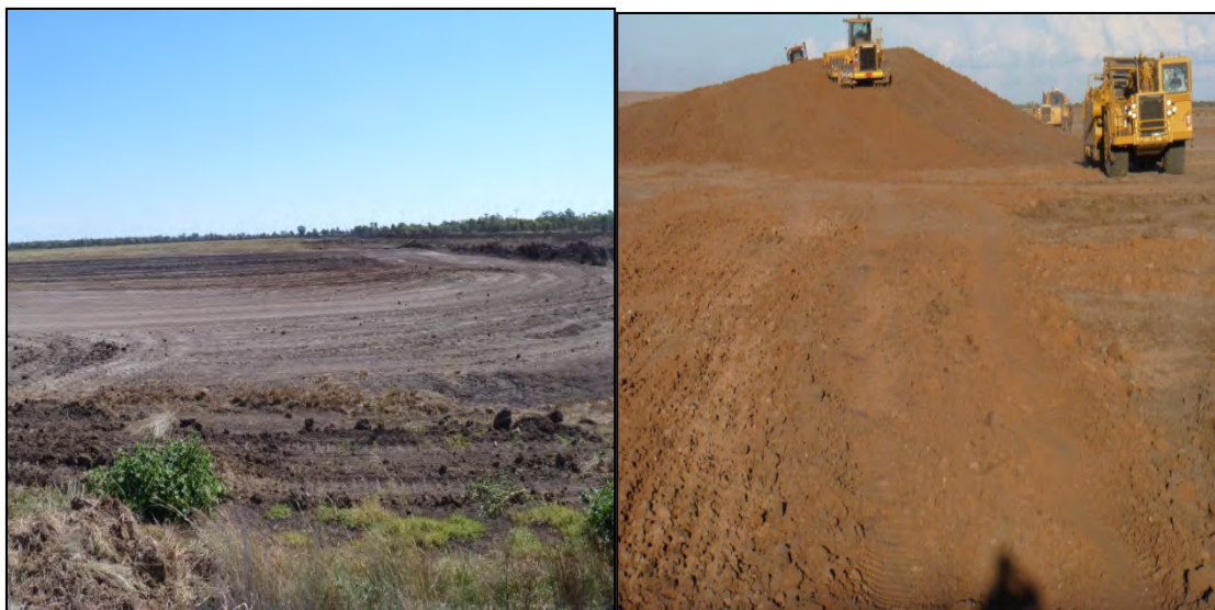
Figure 29: Storage 1 prior to construction (left) and a cross section of the embankment during construction (right).
