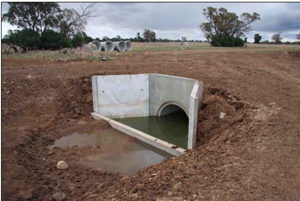
Figure 4: A channel crossing installed on 'Macquarie View' to allow vehicle access and floodwater drainage to pass over the channel.
