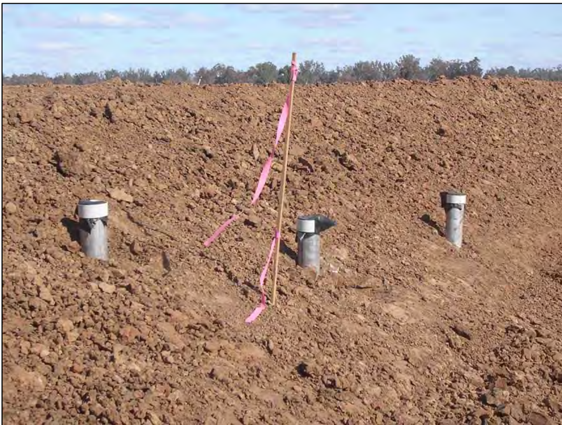
Figure 6: Infiltration tests were conducted as part of the quality assurance program to test the permeability of the compacted clay liner.
