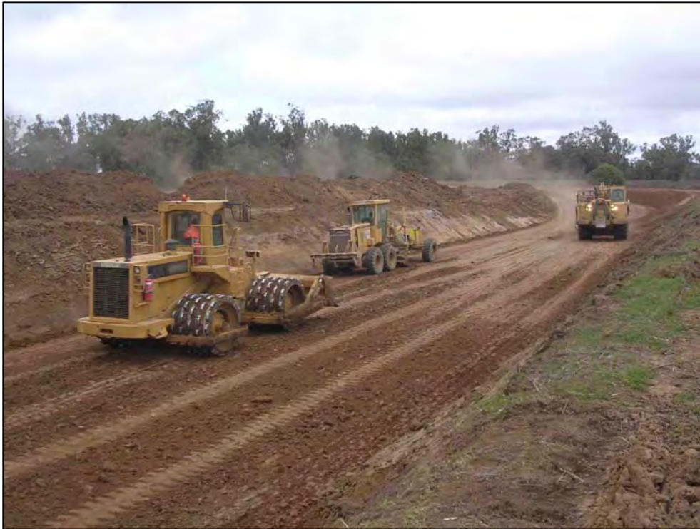
Figure 3: Construction of the new channel linking the Greenhide and Tenandra Scheme. The design included a 0.75 m moisture-conditioned compacted clay lining across the bed of the channel and to a width of four metres under each bank.
