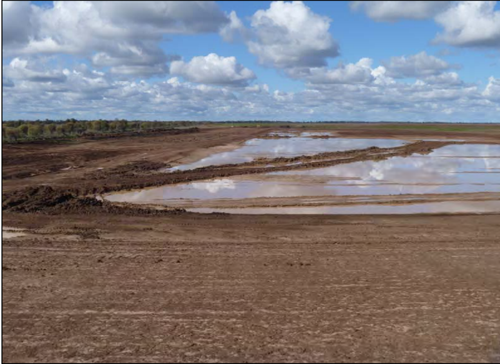
Figure 30: Heavy rain followed by a wetter than normal winter delayed completion of earthworks
