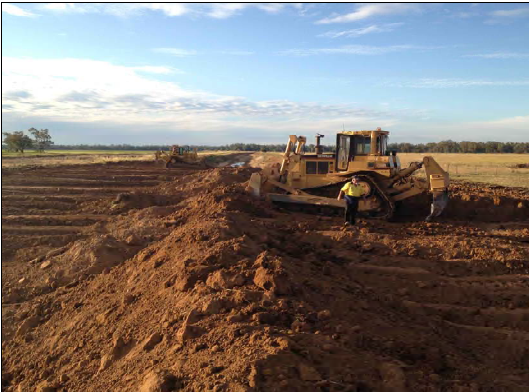
Figure 40: Backfilling operations on a section of decommissioned main channel on ‘Edithville’.
