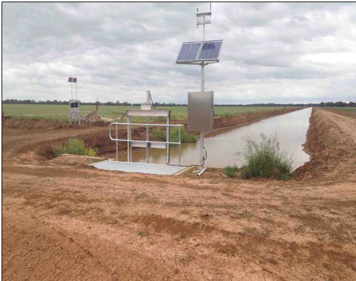
Figure 13: A regulator on ‘Hatton’. Depending on their location, regulators were fitted with single or dual gates, solar-powered electric articulators, Motorola RTU flow measurement, upstream level sensors, gate position sensors and Observant telemetry systems.
