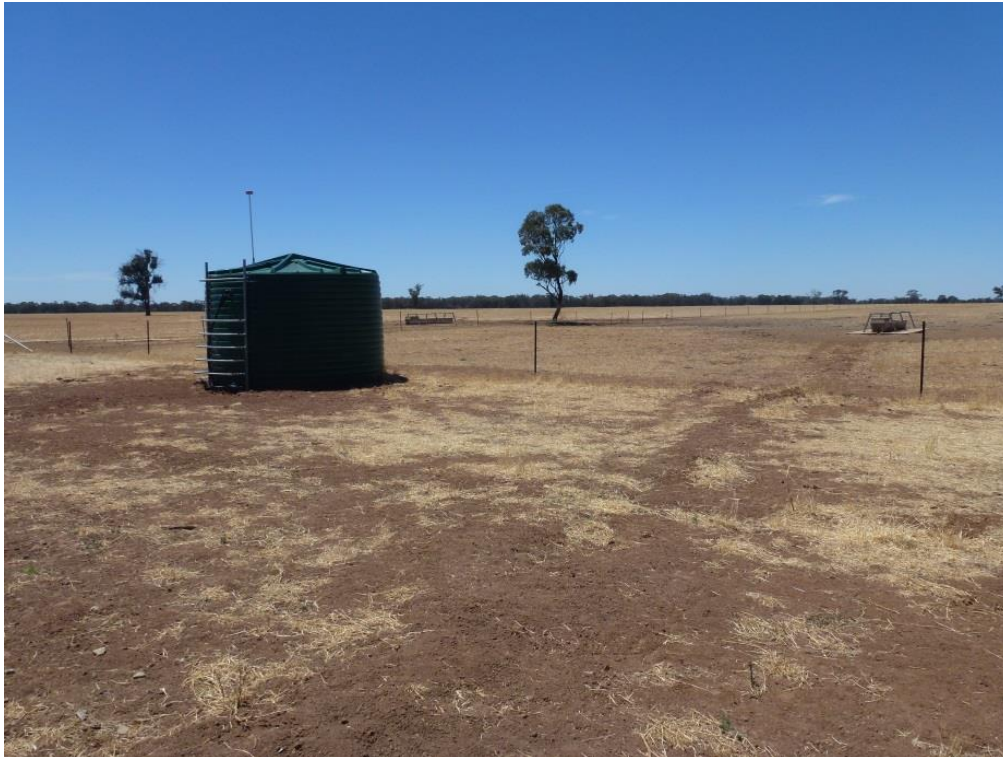
Figure 5: Poly tank with level indicator, guard for inlets/outlets and two water troughs in the background
