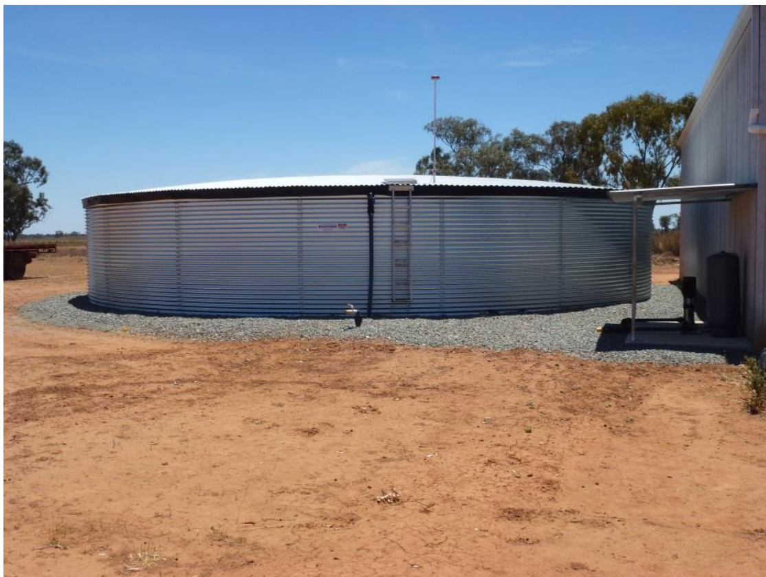
Figure 9: 275 000 litre water tank located at Beverley house with pressure pump to right of photo
