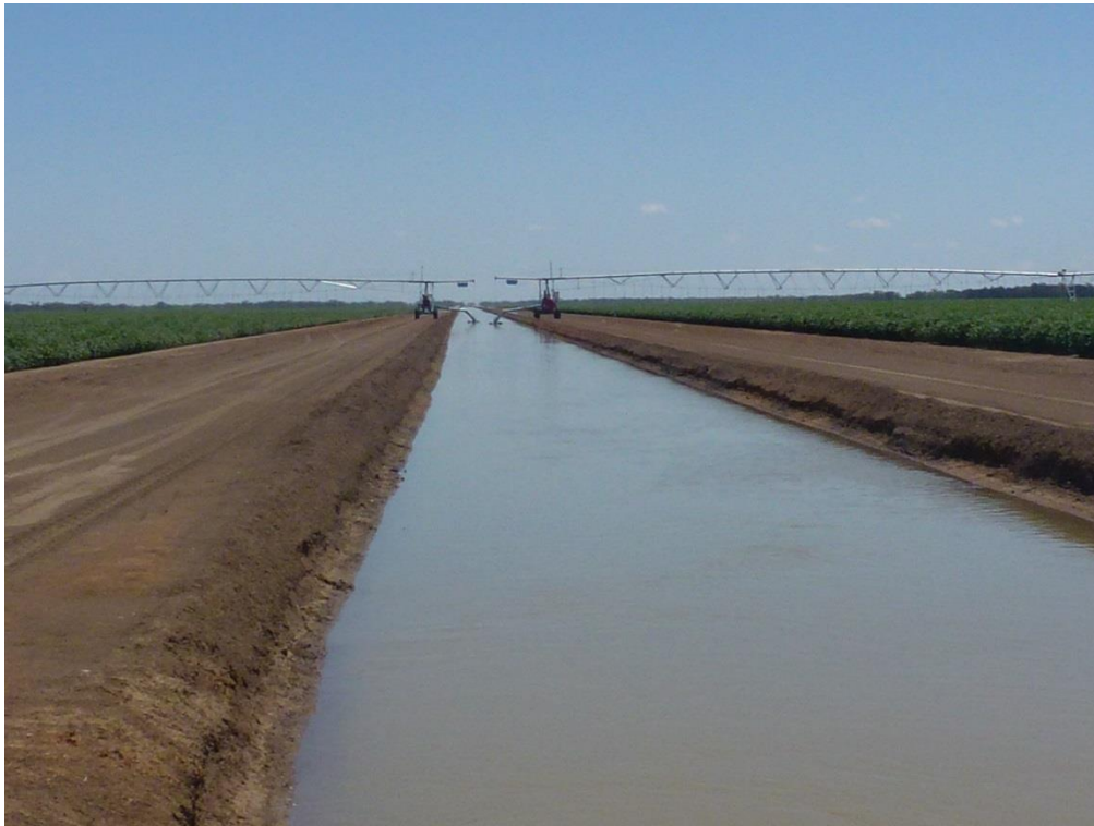
Figure 16: End feed linear move irrigators 2 and 3 showing new supply channel
