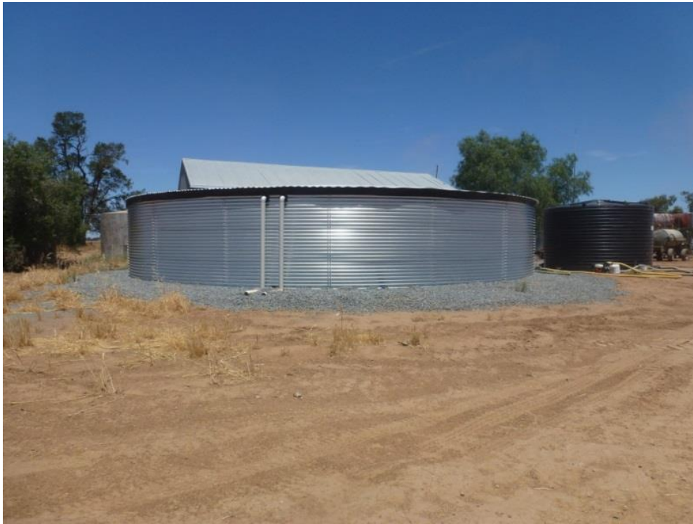
Figure 3: A 275 000 litre steel water tank for storage security
