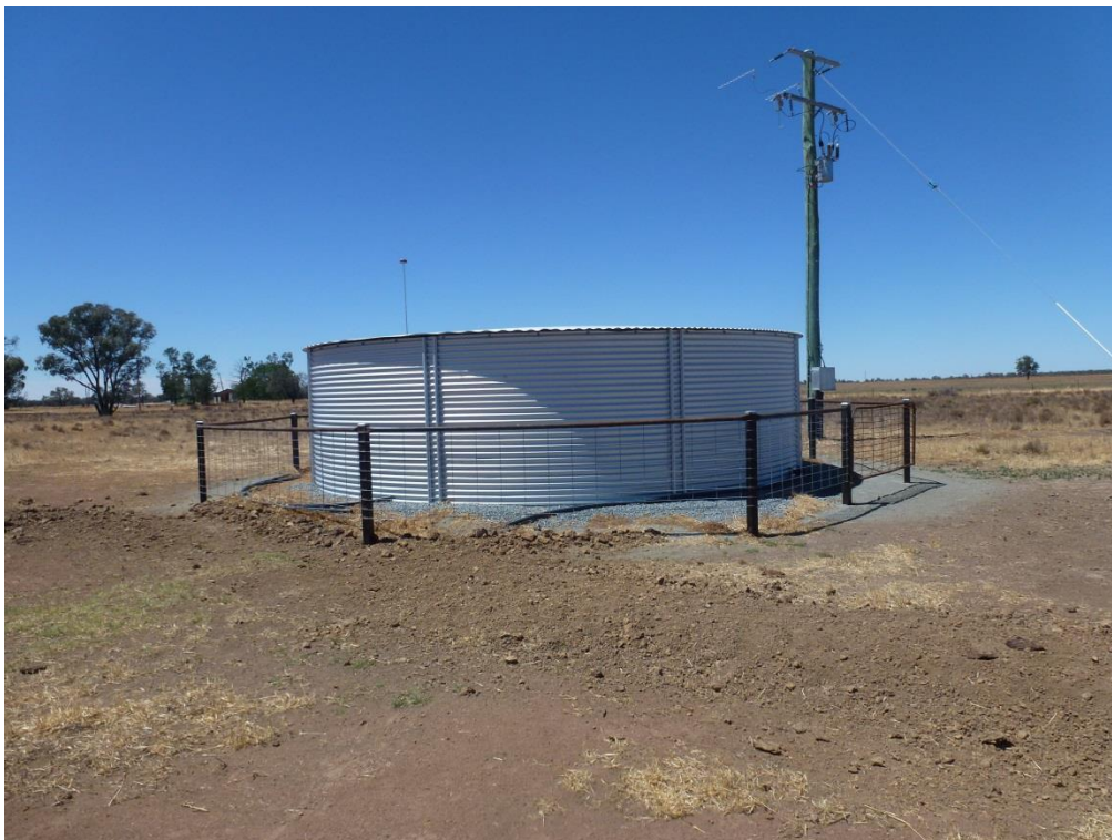
Figure 5s: 100 000 litre storage tank installed on Carroona
