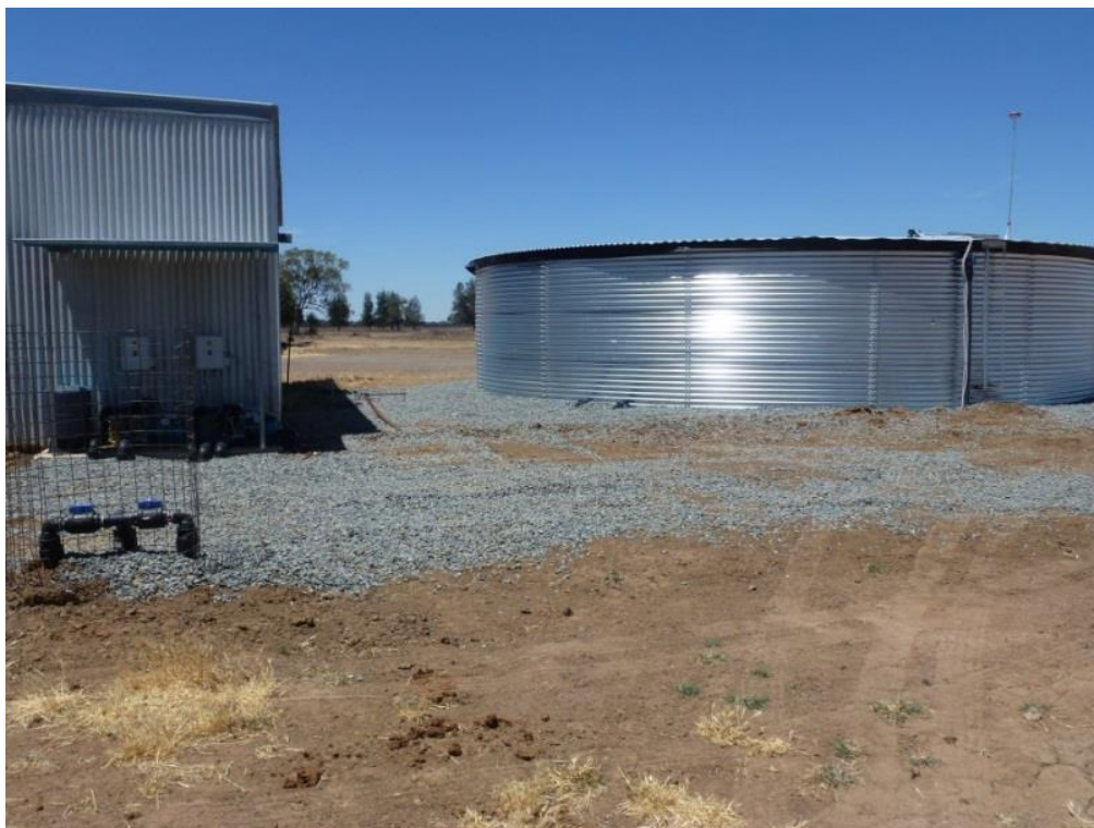
Figure 1: 187 000 litre tank at Gooninbah house
